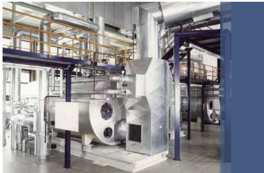
Figure 1: UNIVERSAL steam boiler with ECO 1 Stand-Alone for 1 – 28 t/h steam capacity
