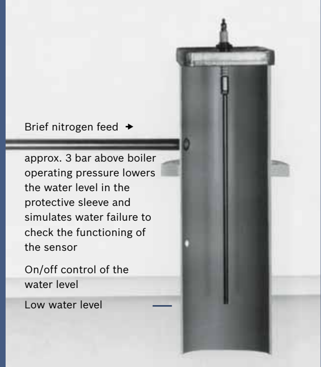
Figure 2: simple electrode – mandatory daily test through blowing in nitrogen.
